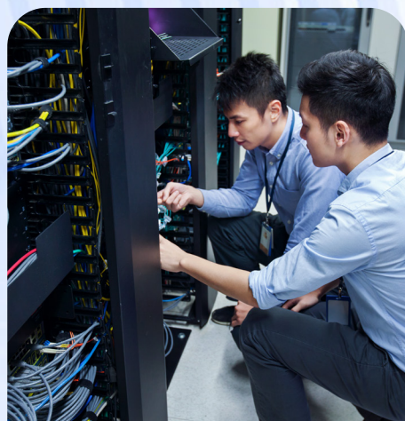
Cable Installation and Maintenance
